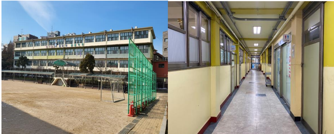
[Fig. 1] Photos of Saebom School: Old Buildings Need to be Rebuilt
