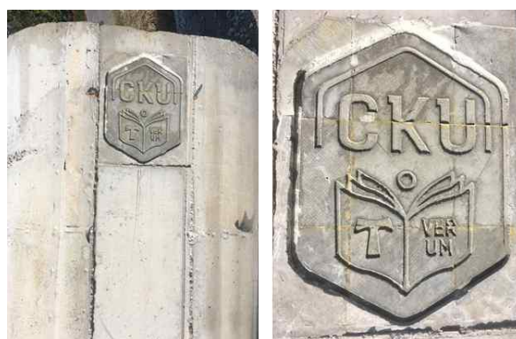
[Fig. 9] Final Logo Clearly Engraved on Concrete Face
