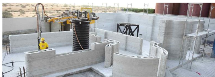
[Fig. 2] 3D Printed Wall Structure for an Administrative Building in Dubai[11]
